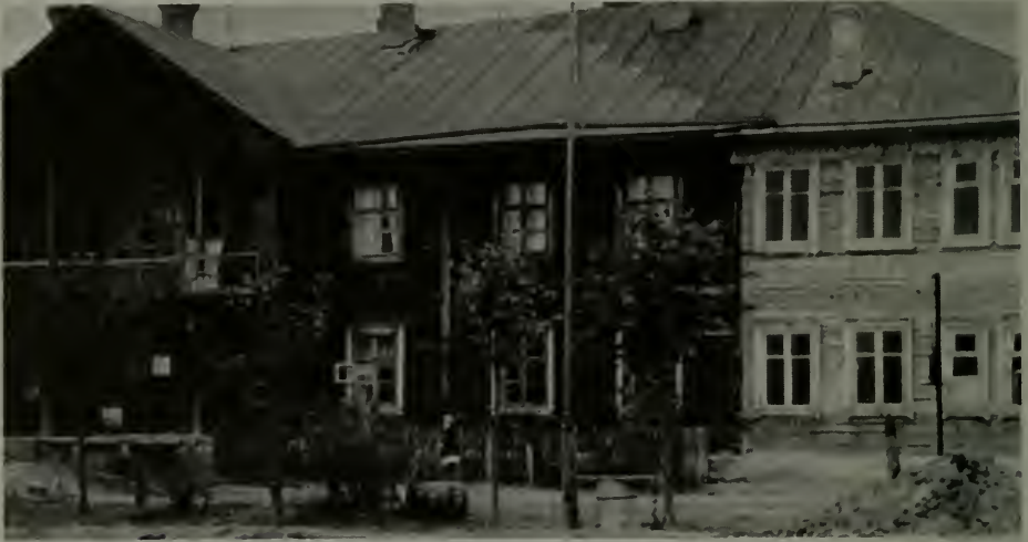
New construction (right) is an addition to staff quarters at Ramensky.
